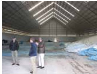
Moulamein Grains Grain Storage Facility
