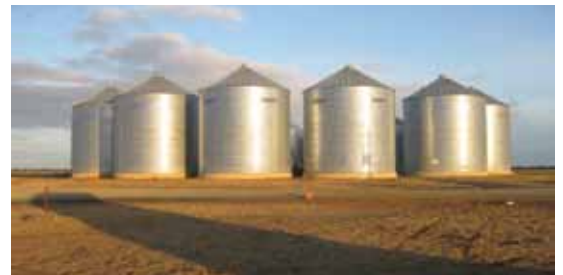
Moama Grains upright silos
